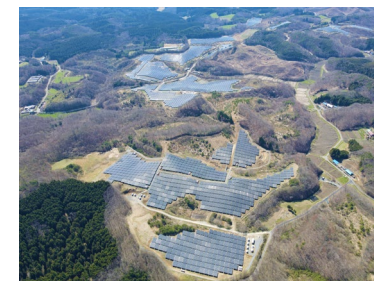
Samegawa Aono Solar Power Plant
