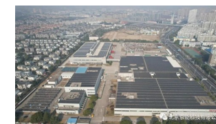
Bird’s-eye view of the SOCC plant
