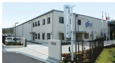
Second plant of Kansai Recycling Systems
