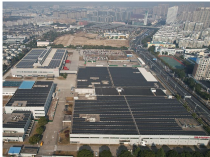
Solar power systems installed on the roofs of Sharp production bases (left: SOCC in China; right: SATL in Thailand)
